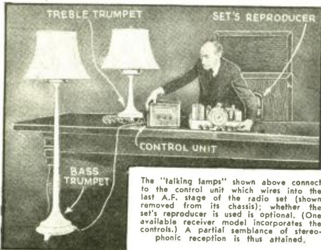
The lamp pedestals are semi-exponential horns. (1255)
